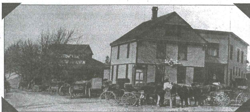
Blanket-covered horses awaited the return of their owners who were doing business in the extensively remodeled premises of August Pump's place, circa 1915, at 5 Corners in the Town of Cedarburg. Pump's buildings, which today comprise the Covered Bridge Inn, included living quarters, saloon, small store and dance hall. Photo courtesy William Malone
