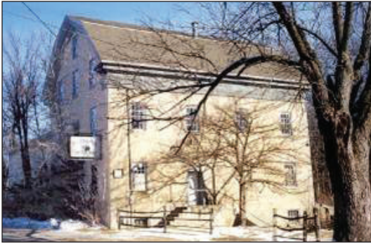
FIGURE 10: Concordia Mill. Source: Town of Cedarburg.
