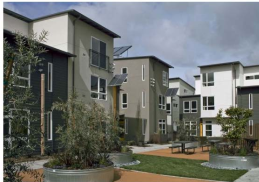
Left: courtyard at a multi-family housing development.
