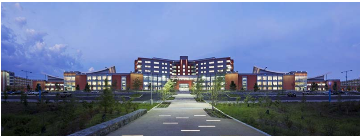
Above: Example of Good Site Lighting
