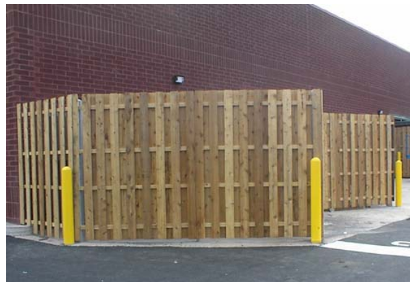
Acceptable Dumpster Enclosures
