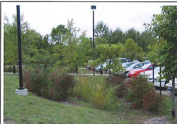
Figure DG 4.5: Rain gardens retain and filter stormwater from parking lots and buildings while existing as attractive landscaping or screening elements
