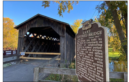
FIGURE 11: Covered Bridge Source: Town of Cedarburg
