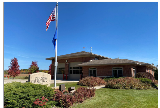
FIGURE 12: Fire Station No. 2 Source: Town of Cedarburg
